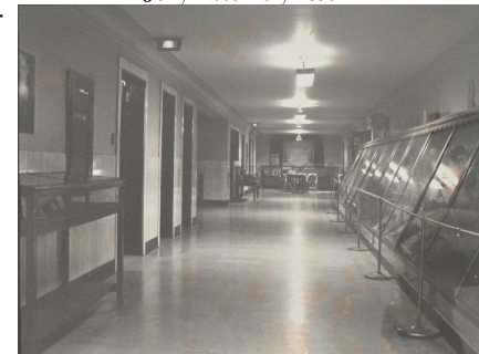
4th floor mezzanine
